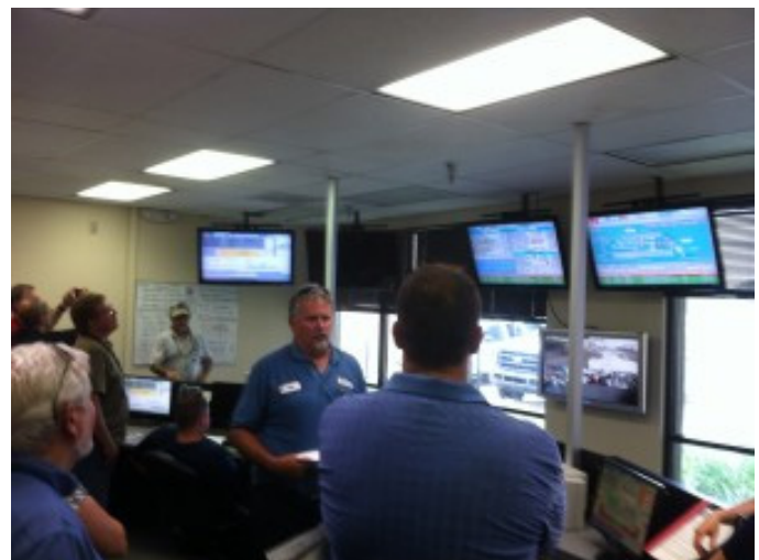
In the plant's new central control room
