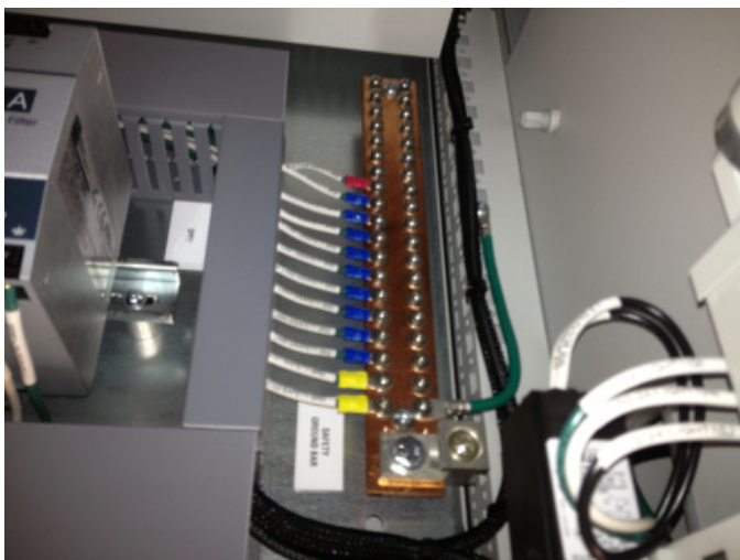
Figure 1- Example Ground Bar in a Control Panel
